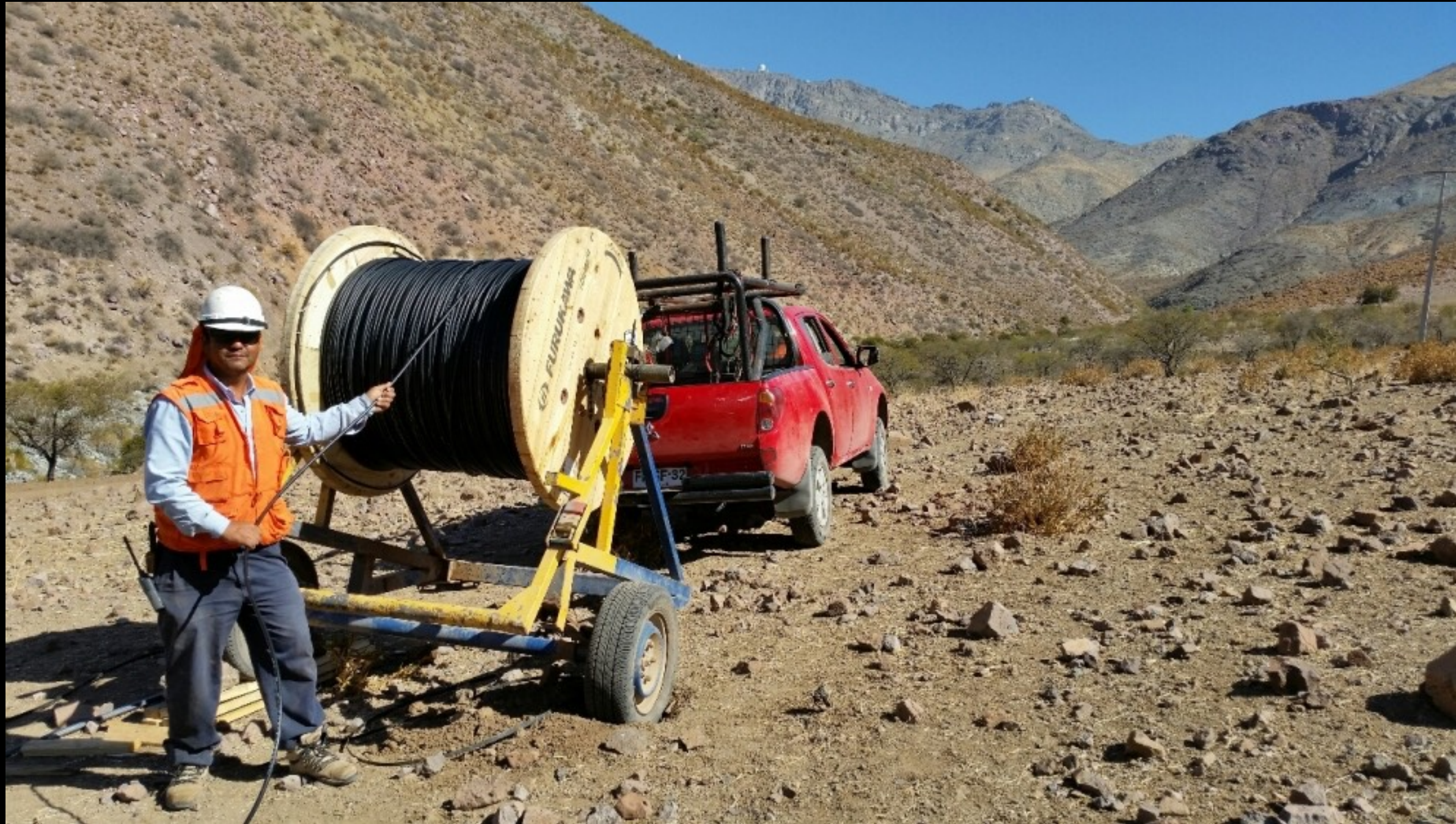
Laying fiber optical cable from summit
